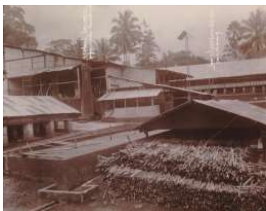
Figure 7. Construction of a rubber factory, coffee drying house. the Kali Klattak company in Klatak Banjoewangi in 1925 (Source: kitlv.nl)
