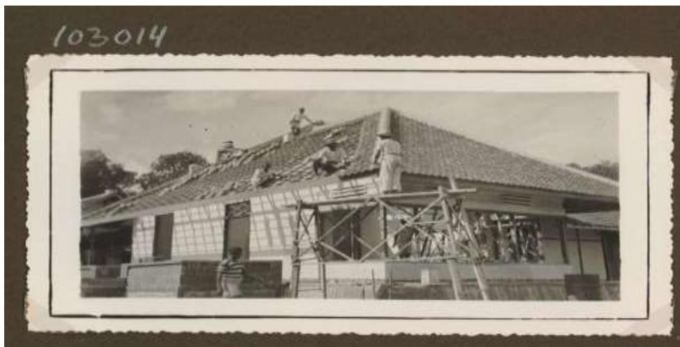
Figure 10. Renovation of the official residence of the Kali Klattak plantation administrator in Klatak Banjoewangi in 1925 (Source: kitlv.nl)
