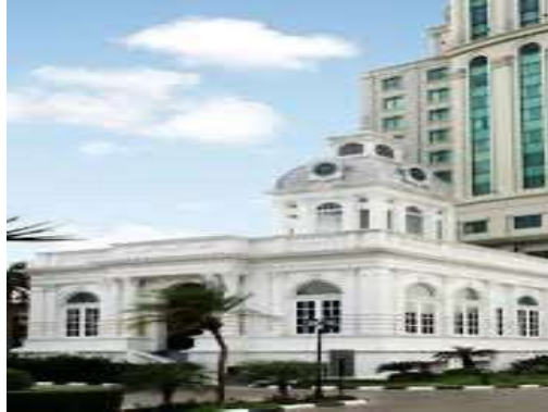
Gambar 2: City Hall Building
