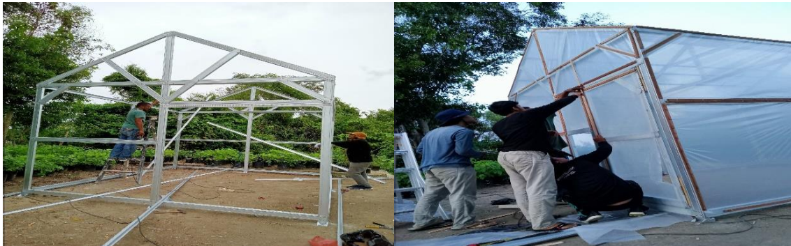
Figure 4. Greenhouse Construction Process Using Steel Frame Material.
