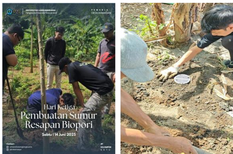
Figure 1 Biopore Infiltration Well Construction Activity
