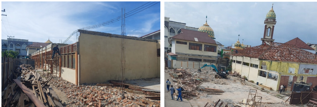
Figure 1. Existing Condition of the DPIB Laboratory Building and Its Surrounding Environment at SMK Negeri 5 Padang
