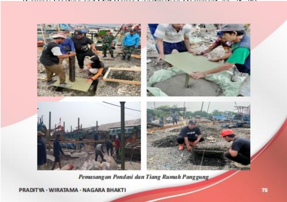
Figure 2. Installation of Foundations and Pillars of a Stilt House (Source: Floating and Stilt House Construction Document, p. 75)
