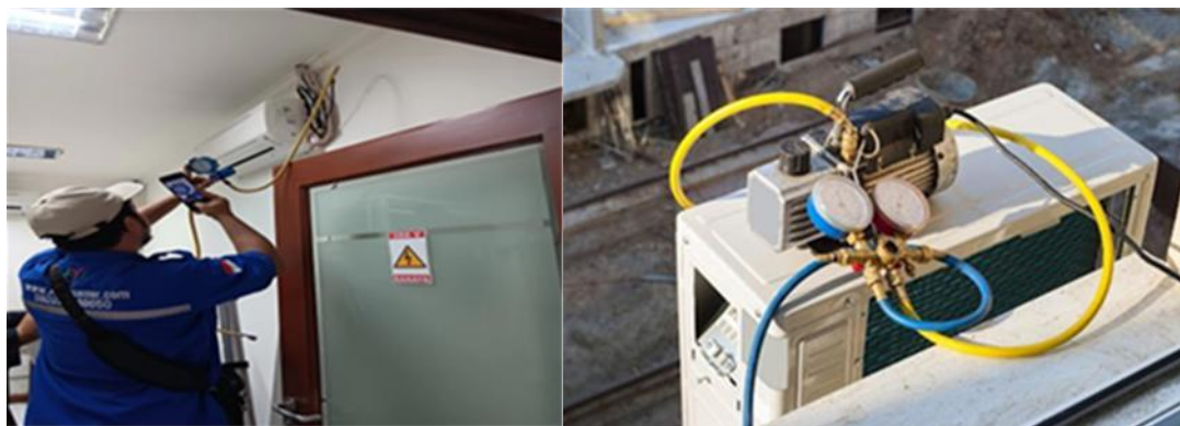
Figure 5. Refrigerant Checking and Filling
