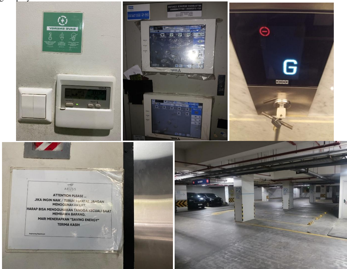
Figure 4. Environmental Facilities Supporting Green Hotel Practices
