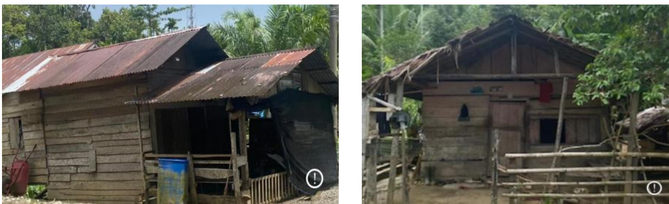
Figure 2. Exterior view of RTLH in Panton Reu District
