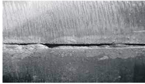
Figure 1. Undercut in Welding
