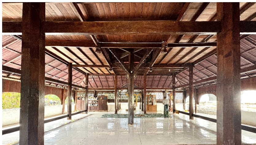
Image 4. Timber columns and upper structural rhythm in the prayer hall
