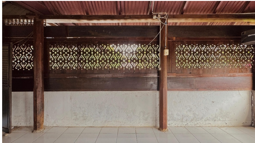
Image 3. Wall composition with solid base, timber panels, and perforated ornament
